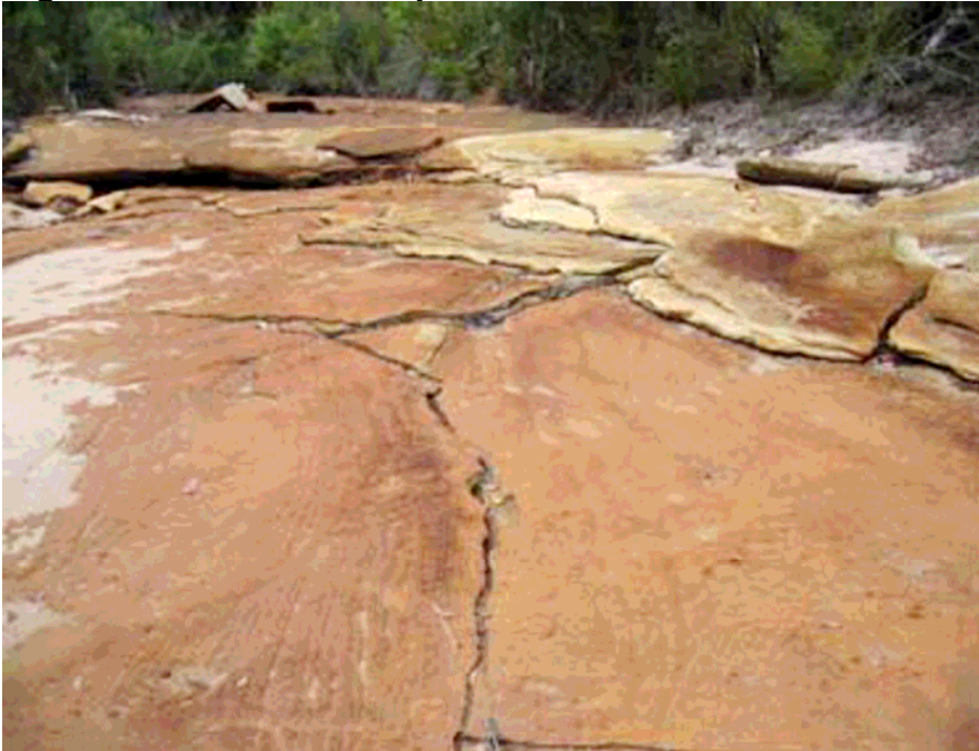
Figure 5: Subsidence Impacts at Waratah Rivulet
